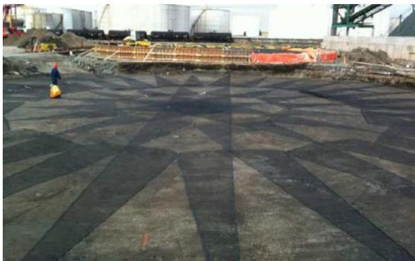
a) Geogrid reinforcement on excavation base
