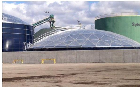
b) Tank built on geogrid-reinforced ground mass
