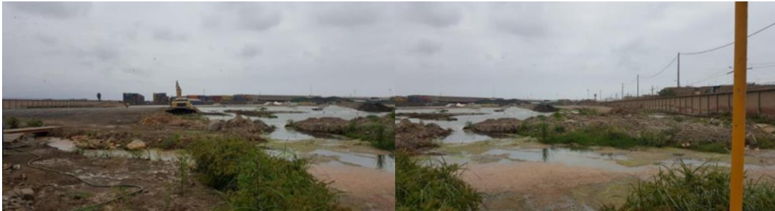
View of the conditions of the foundation land
