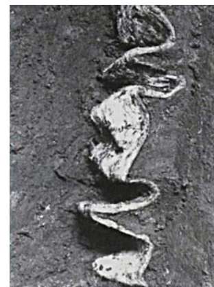
Fig. 2 Buckling of drain material due to large relative compression of the ground (Cortlever and Hansbo 2004)
