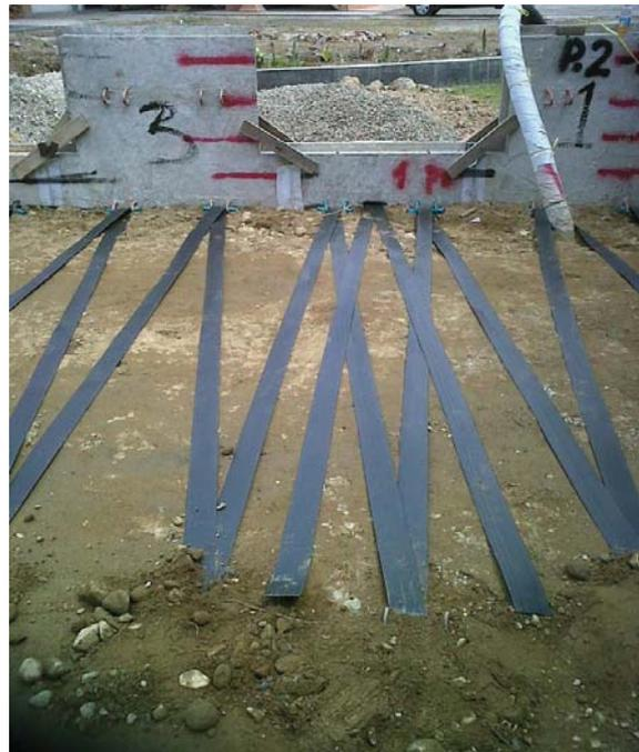
Fig. 1 Field installation of MSEW with anchored V-configuration polyester straps.
