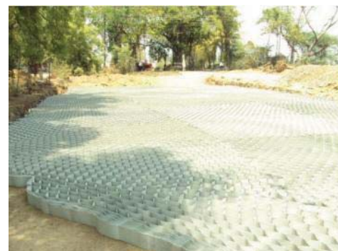
Fig. 3 Geocell layer spread over the road section
