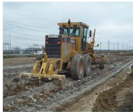
Fig. 2 Mixing of the lime by a tractor
