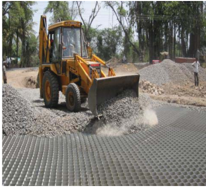
Fig. 4 Filling the geocell pockets
