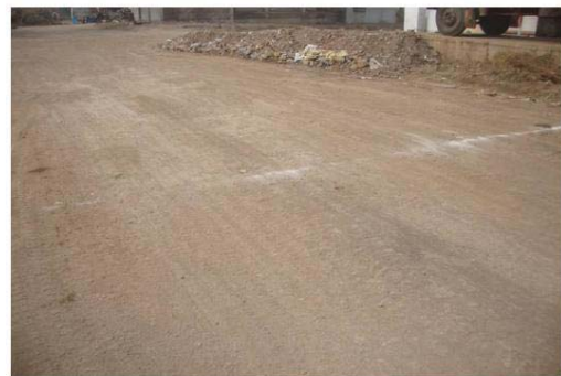
Fig. 7 Geocell reinforced pavement with uniform surface
