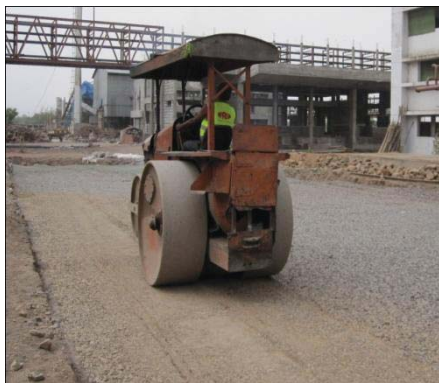
Fig. 5 Compaction by a vibro roller
