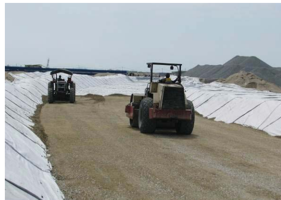
Fig. 9 Compaction of crusher run
