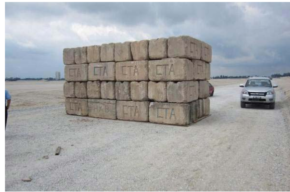
Fig. 13 Maintained load test
