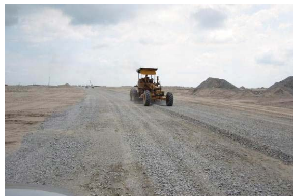
Fig. 10 Leveling the final layer of crusher run
