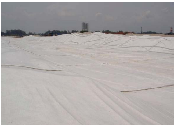
Fig. 7 Laying of second layer of reinforcement
