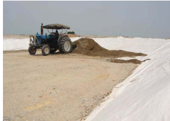
Fig. 8 Laying of crusher run
