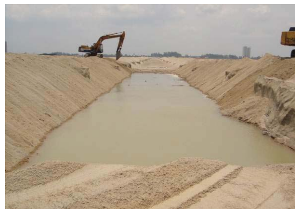
Fig. 5 Excavation of loose sand
