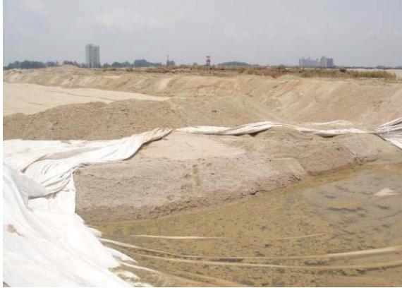
Fig. 6 Laying of the first compacted layer reinforced with geotextile
