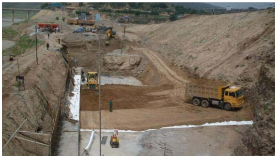
Fig. 10 Laying of initial reinforcement layer over prepared surface
