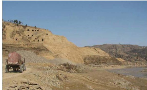
Fig. 3 Hill slope with cave dwellings at Hetaoyu project site
