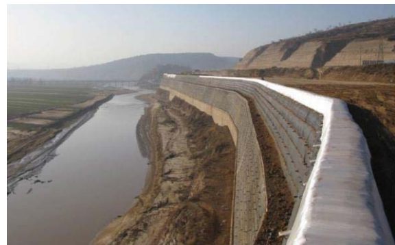
Fig. 12 View showing wraparound of reinforcement geotextile over soil bags
