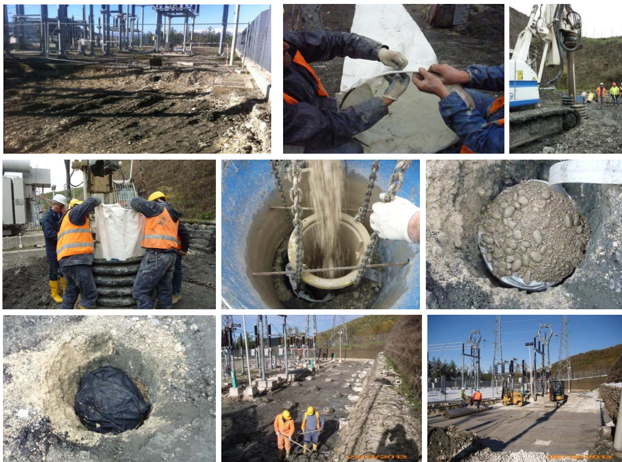
Figure. 7. The construction sequence (from right to left and top to bottom): excavation up to desired level; fixing the circular steel loop to tubular geotextile; excavation with drilling machine; lowering GEC in the drilled hole; filling through hopper; filled column; covering end of column with nonwoven geotextile; rows of completed GEC; placing the GCL on top of GEC.
