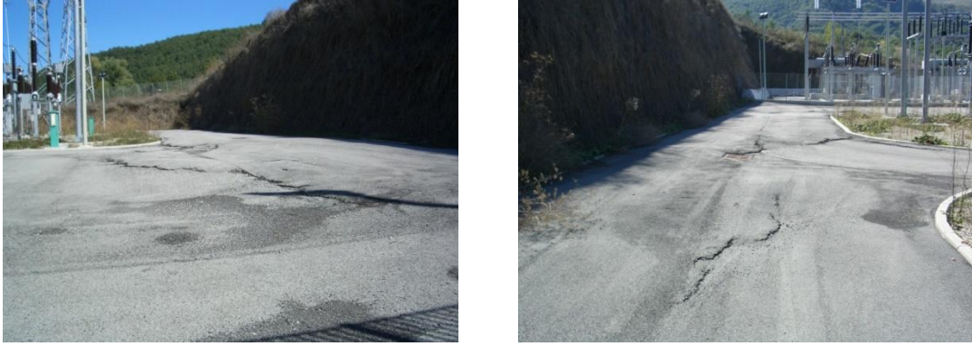
Figure. 3. Heave of the pavements of the yard in the electrical substation (SSE) of Monteferrante
