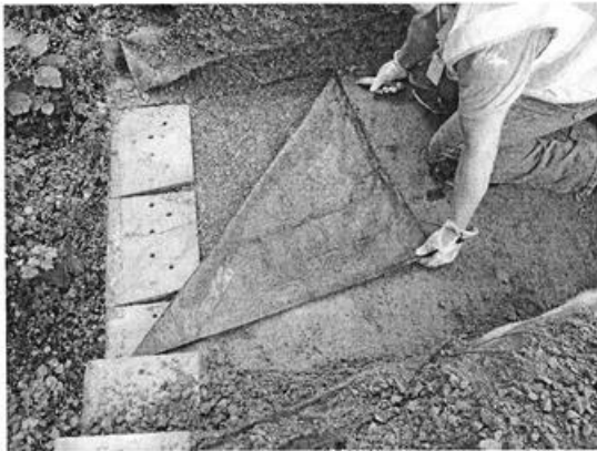
Figure 5. Cutting away the geotextile
