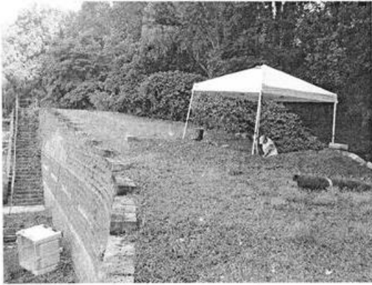
Figure 3. Overview of the work site
