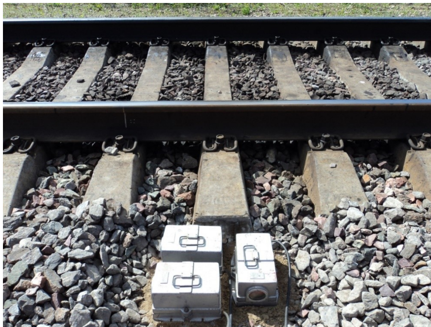
Figure 6. Preparation of test site.
