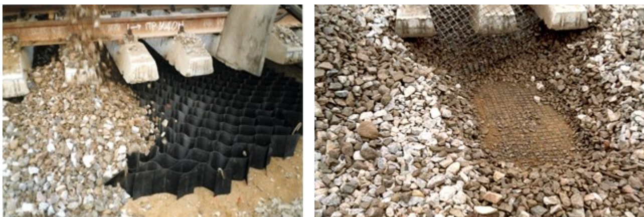
Figure 4. Laying of geocells and two geogrid layers.
