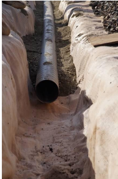
Figure 3: Installation of the geosynthetic clay liner in the infiltration ditch
