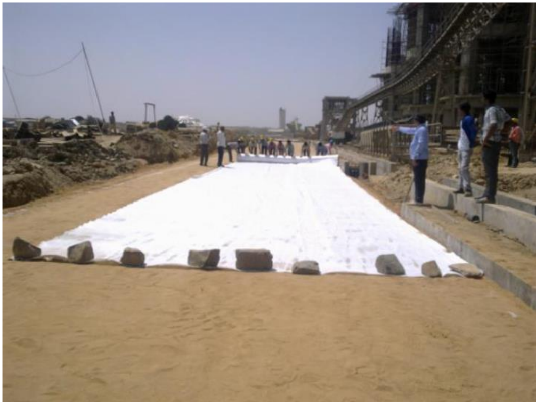
Figure 4. Laying of Non-woven geotextile.
