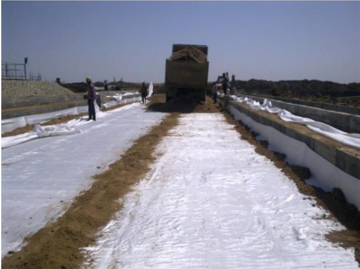
Figure 7. Sand layer placement over woven polyester geotextile.
