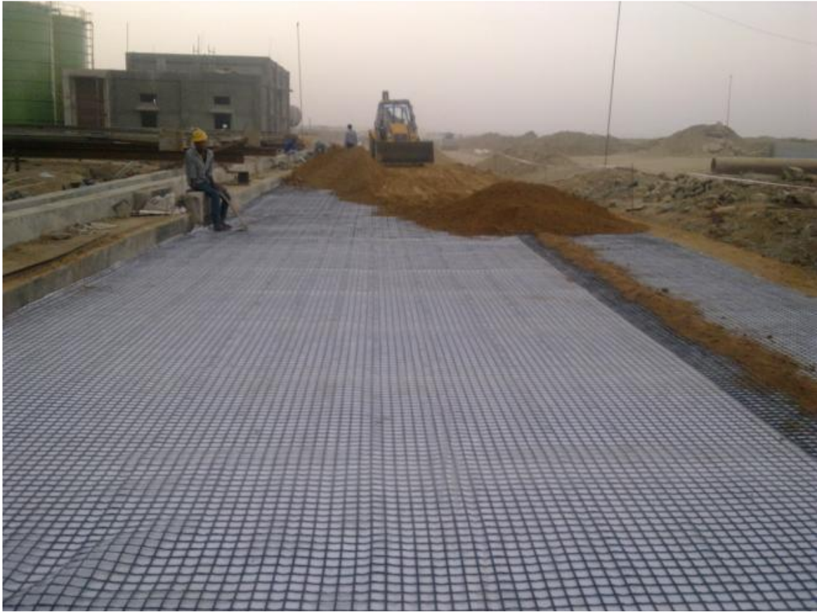
Figure 6. Sand layer placement over geogrids.
