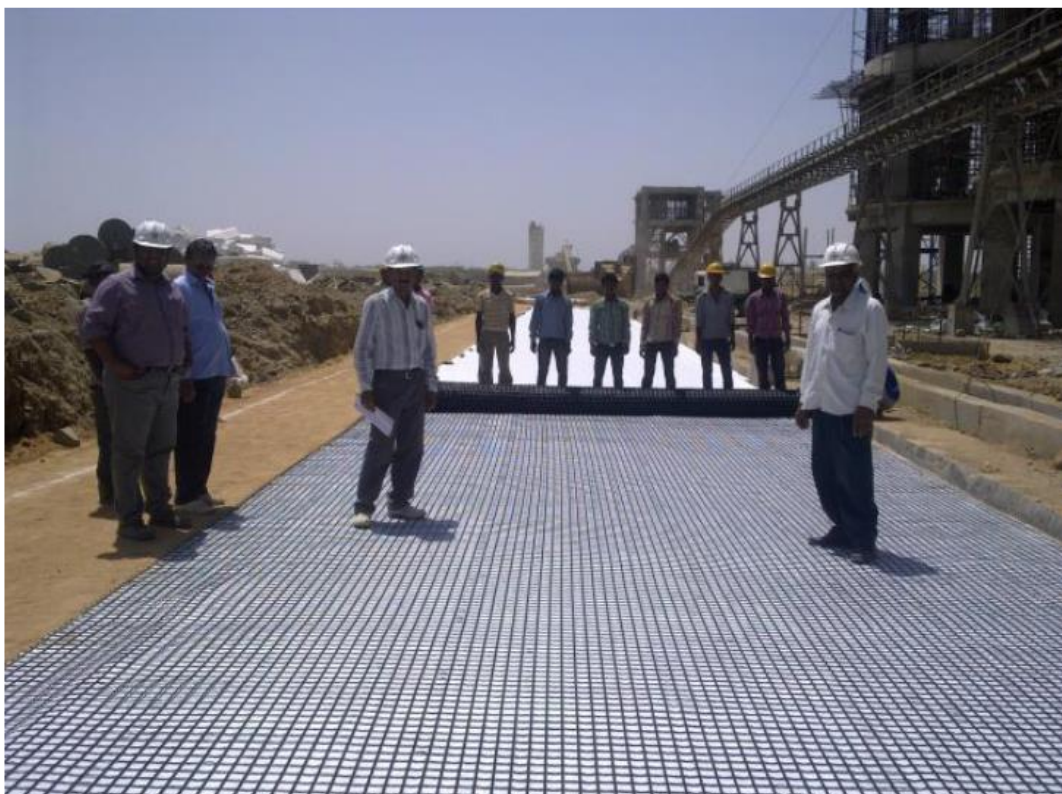
Figure 5. Laying of bi-axial geotextile over non-woven geotextile.
