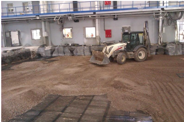
Figure 9. Works at upper most layer (a) fill placement, (b) compaction.
