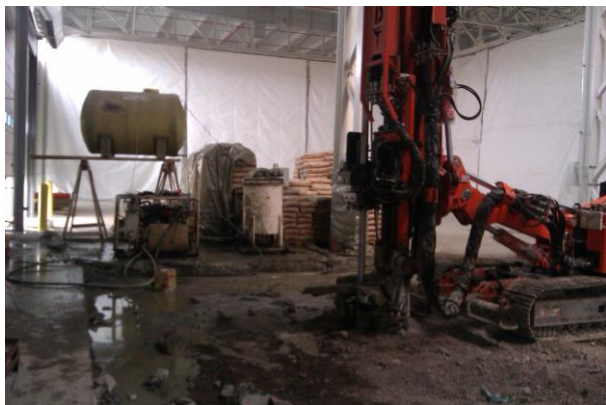
Figure 6. Jetgrout application
