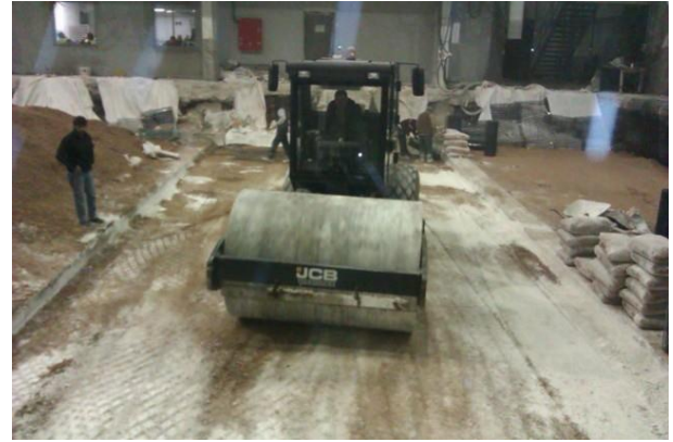
Figure 8. Lime stabilization
