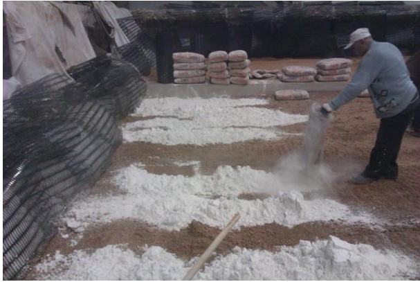
Figure 8. Lime stabilization
