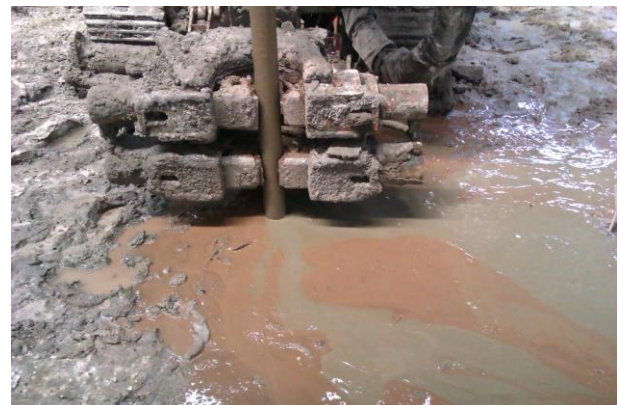
Figure 6. Jetgrout application
