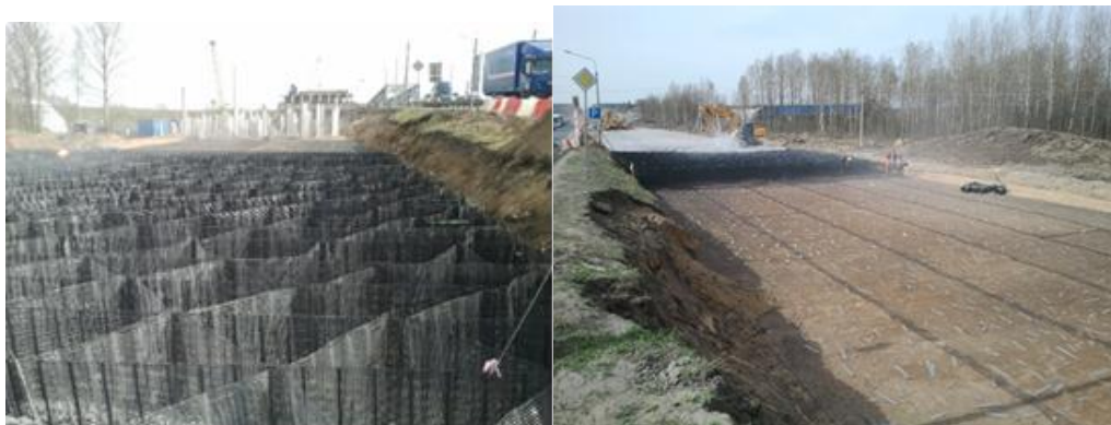
Figure 4. Geocell mattress installation.
