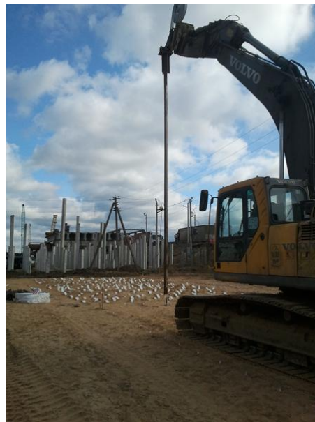
Figure 3. Drains installation
