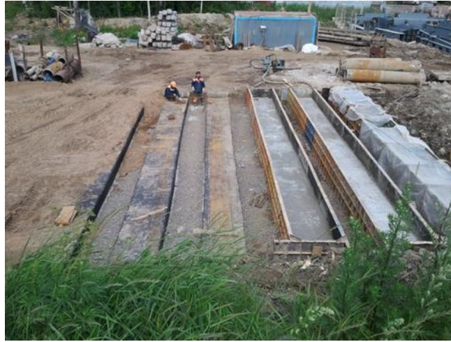
Figure 2. The grid foundation
