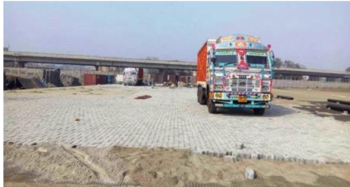
Figure 4(d). Completed paving with geocells
