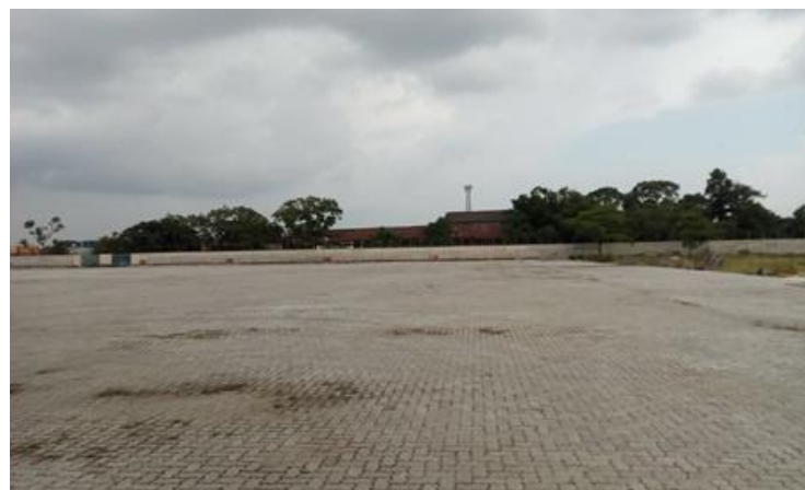
Figure 5. Completed paving with geocells after one year
