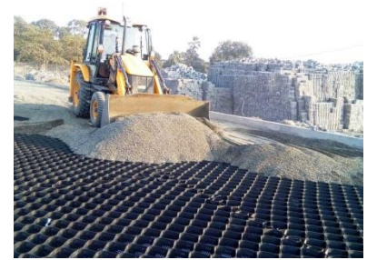
Figure 4(c). Infilling of geocells
