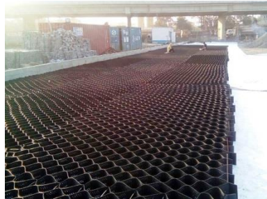
Figure 4(b). First layer of geocells laid over nonwoven
