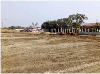
Figure 4(a). Dressed fill surface
