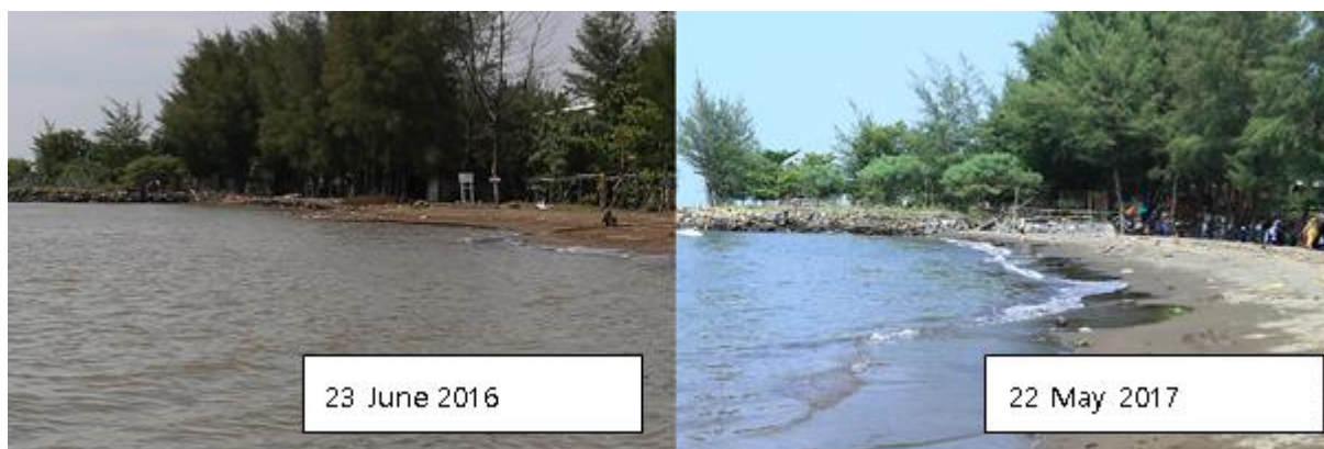
Figure 8. the coast line is refilled with sand
