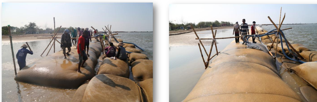
Figure 7. The result of geotextile tube
