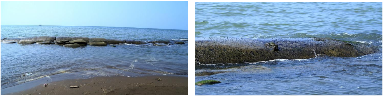
Figure 9. The geotextile tube after 12 months of installation
