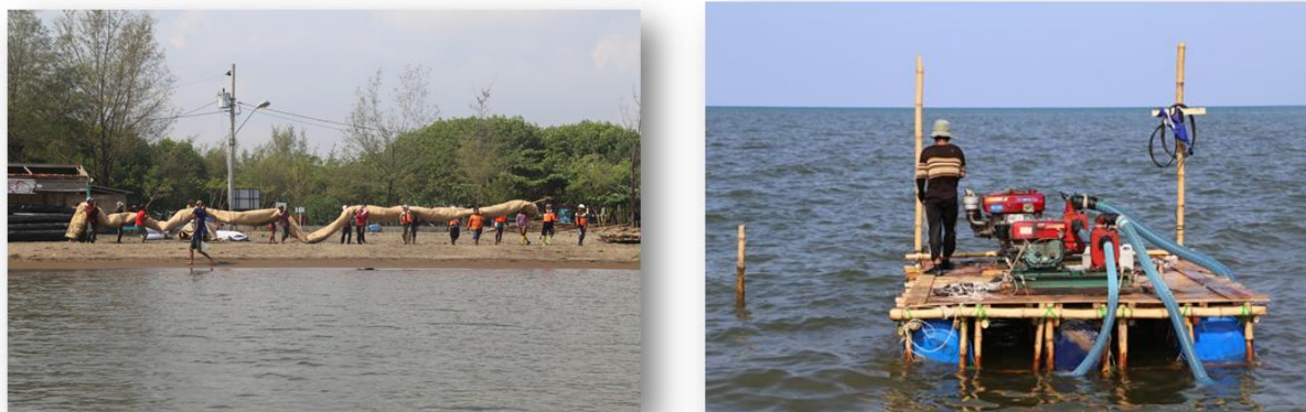
Figure 6. construction of geotextile tube
