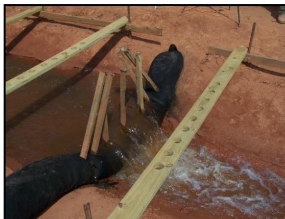
Figure 10. Testing of a Compost Sock
