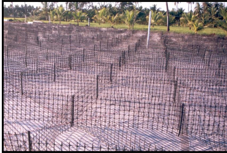
Figure 4. A view of the 1 m high geocell mattress prepared
