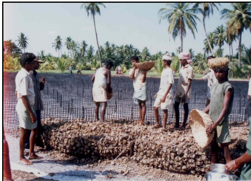
Figure 5. A view of filling the cells with stones
