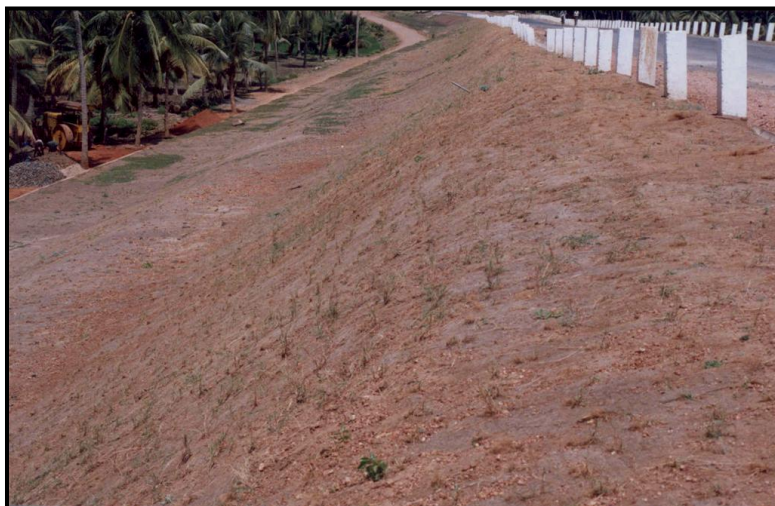
Figure 7. A completed view with erosion control blanket
