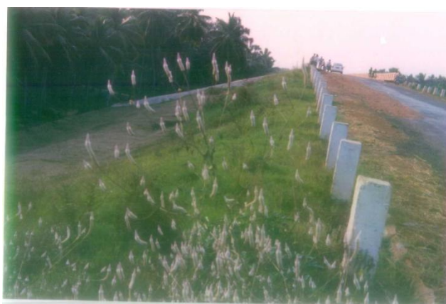
Figure 8 The embankment of a monsoon season, with profuse growth of turfing.
