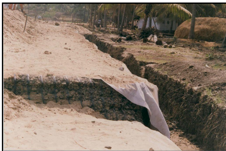
Figure 6. A view of the non wovengeotextile enveloping the geocell mattress
