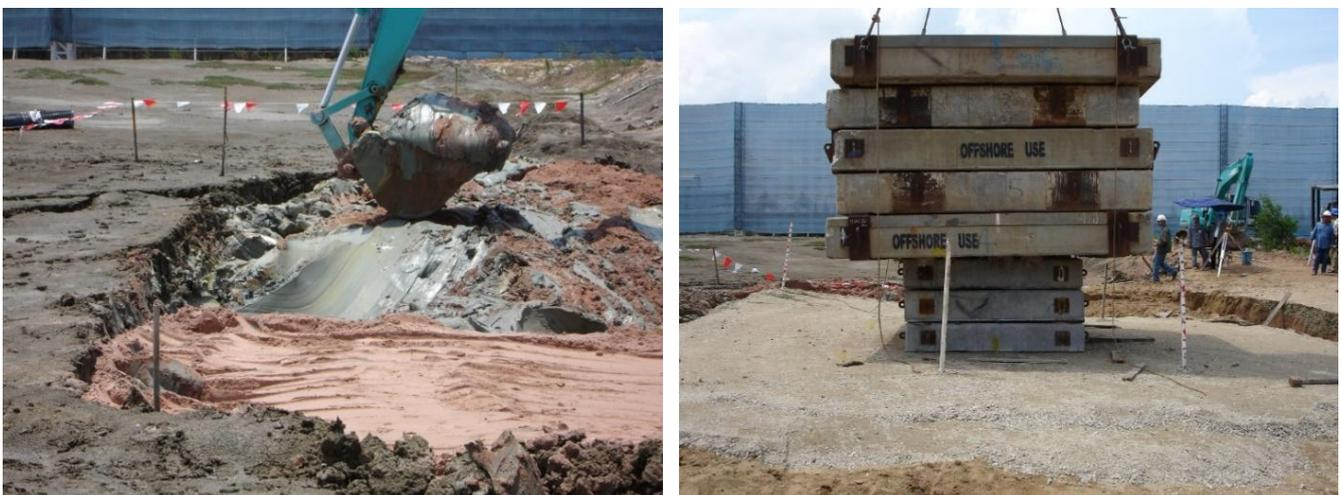
Figure 4. Laem Chabang fabrication yard: initial ground conditions (left) and final load test arrangement (right)
