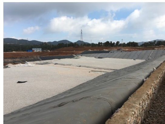
Figure 4 Job site overview
