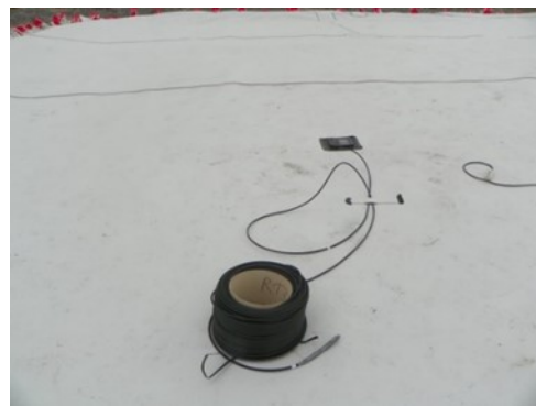
Figure 17 Combi-Module embedded in leak location liner Figure 18 Combi-module and cable wire after installed
