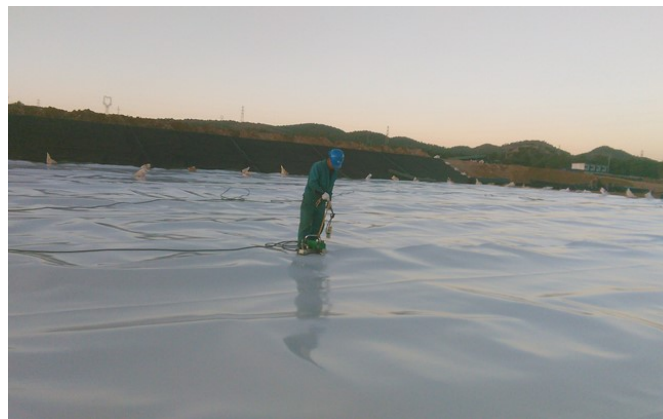
Figure 8 Leak location liner field welding in progress
