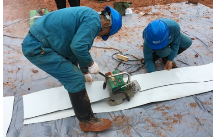
Figure 7 Iso-Wedge trial welding
