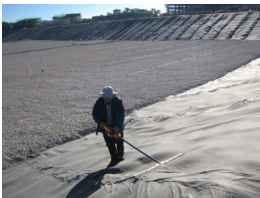
Figure 9 Spark testing at slopes
