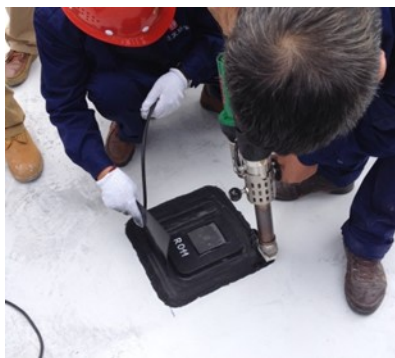
Figure 17 Combi-Module embedded in leak location liner Figure 18 Combi-module and cable wire after installed
