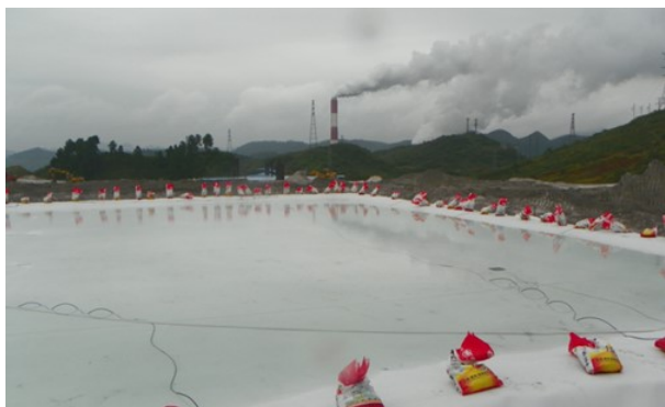
Figure 20 Test pad flooded with acid water
