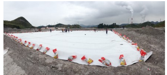
Figure 13 Overview after liner installation
