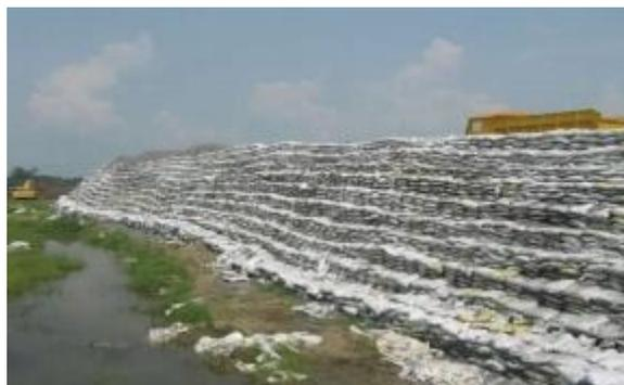
Figure 9: Pre-loading with flyash, height – 10m
