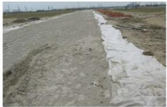
Figure 8: Geotextile separator
