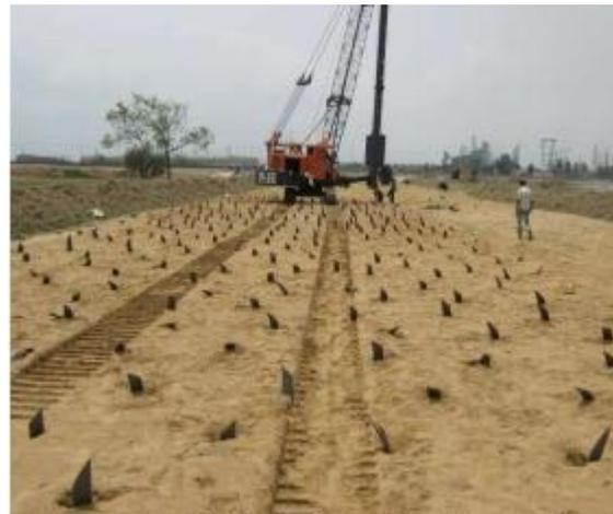
Figure 4: Installation of PVD in Site (Plan)
