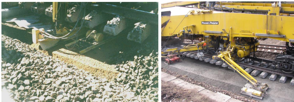
Figure 4. Ballast cleaning machine SCHU-800 and track machine AXM 800.
