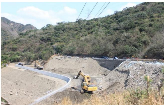
(a) Construction of pile-supported protection wall.
