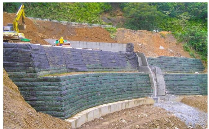
(b) Construction of reinforced earth slope.
