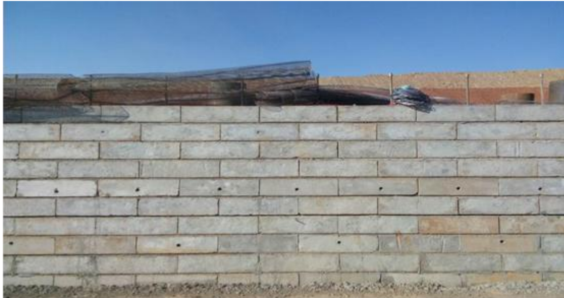
Fig.2.1 The wrap-styled reinforced earth retaining wall
