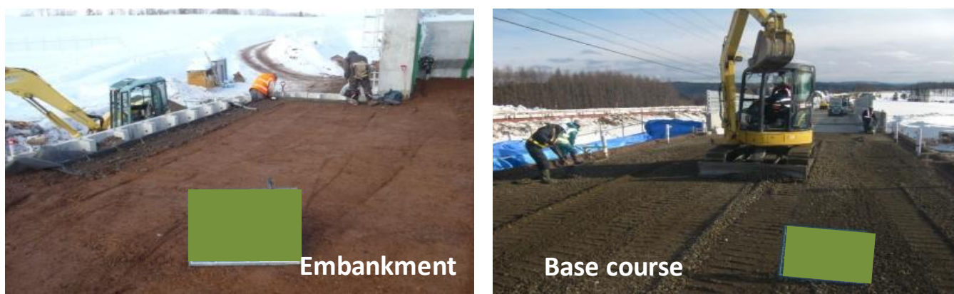
Figure 2. The embankment and the base course under construction.
