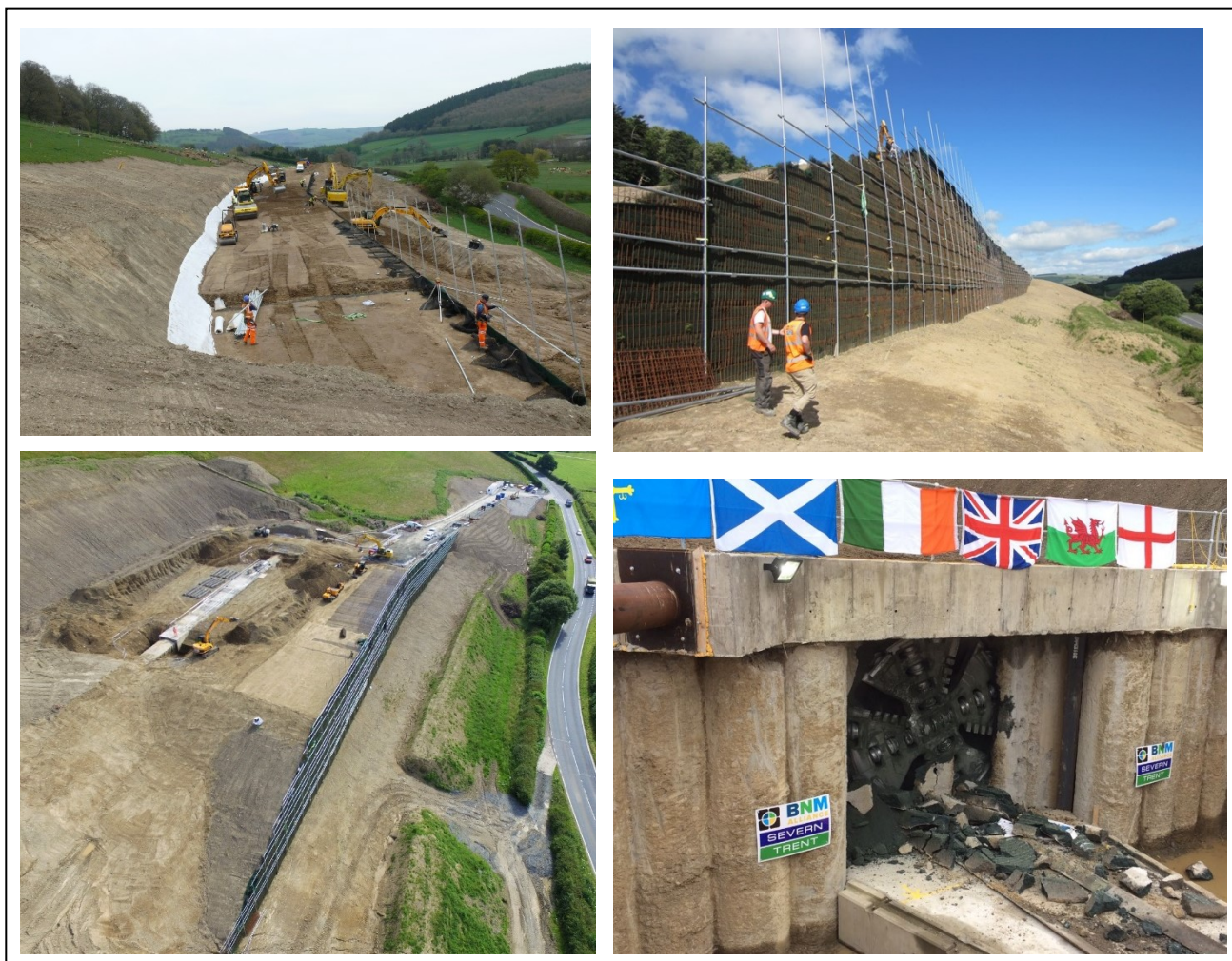
Figure 8. RSW Construction process and breaking through TBM – Elan Valley Bleddfa
