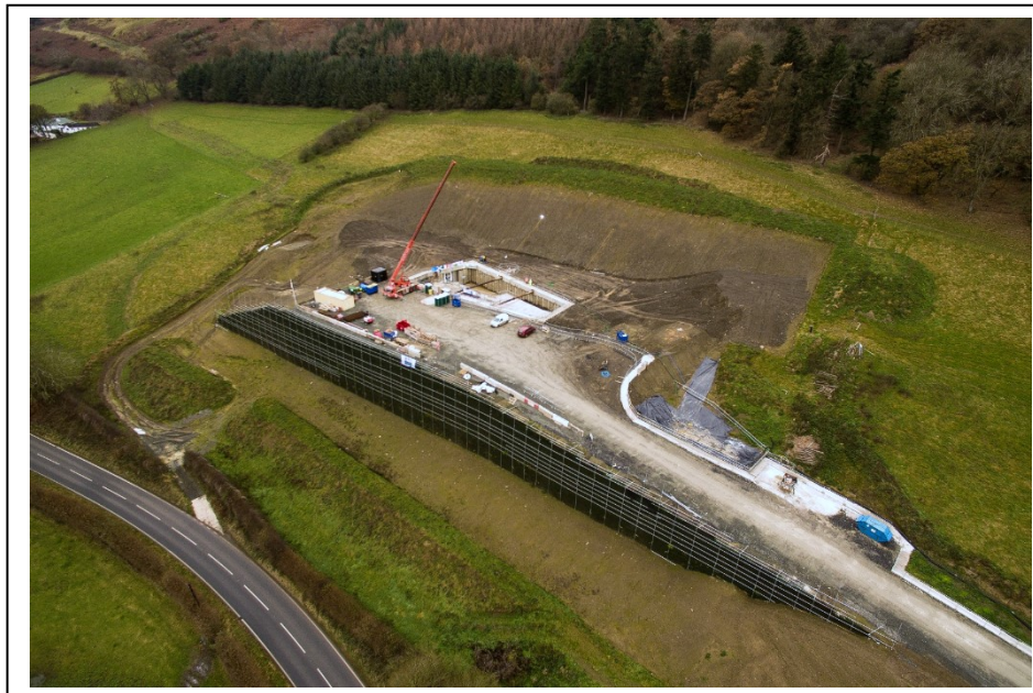
Figure 2. Aerial View: Construction of RSW EVA Bleddfa
