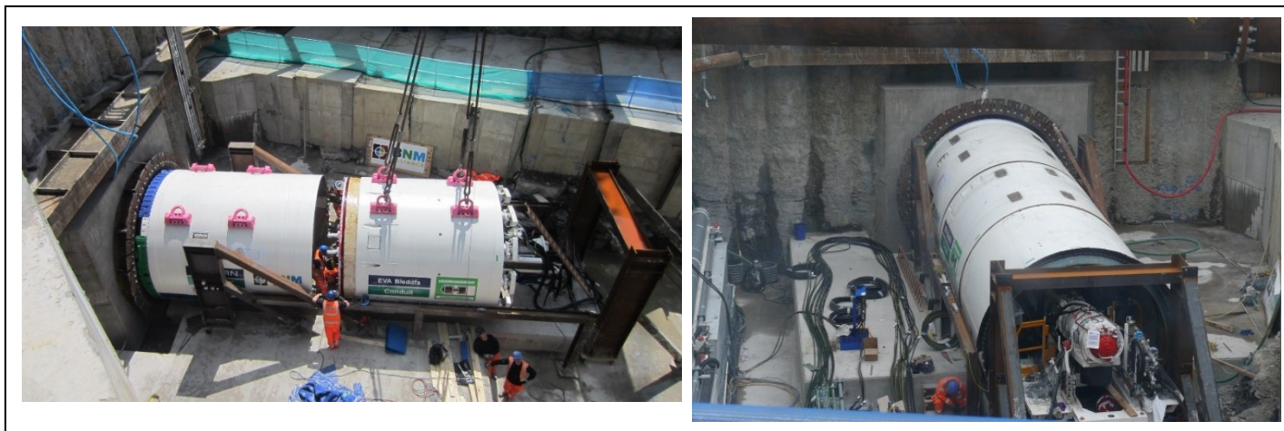
Figure 4. Tunnel Boring Machine TBM (150 ton)
