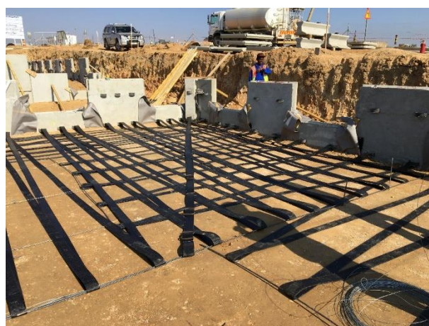
Figure 7: Paraweb reinforcement installed
