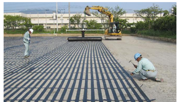
Photo 2. Installation status of geosynthetics
