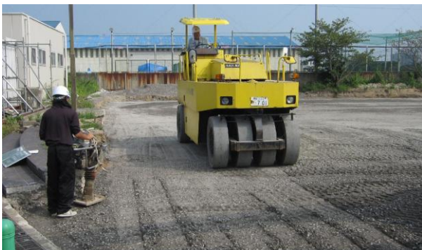
Photo 1. Compaction status of gravel layer
