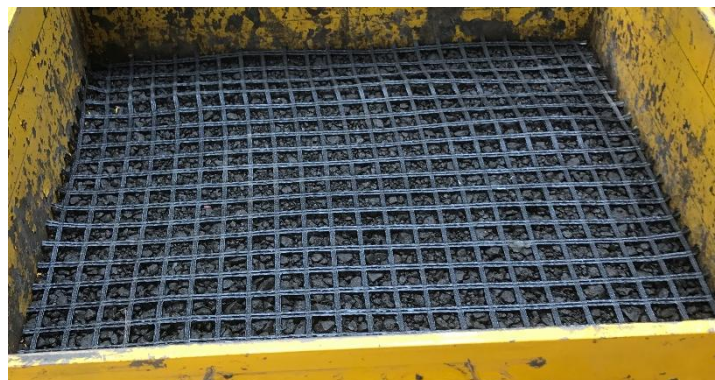
Figure 9. Polymer Geogrid Placed at RAP Base
