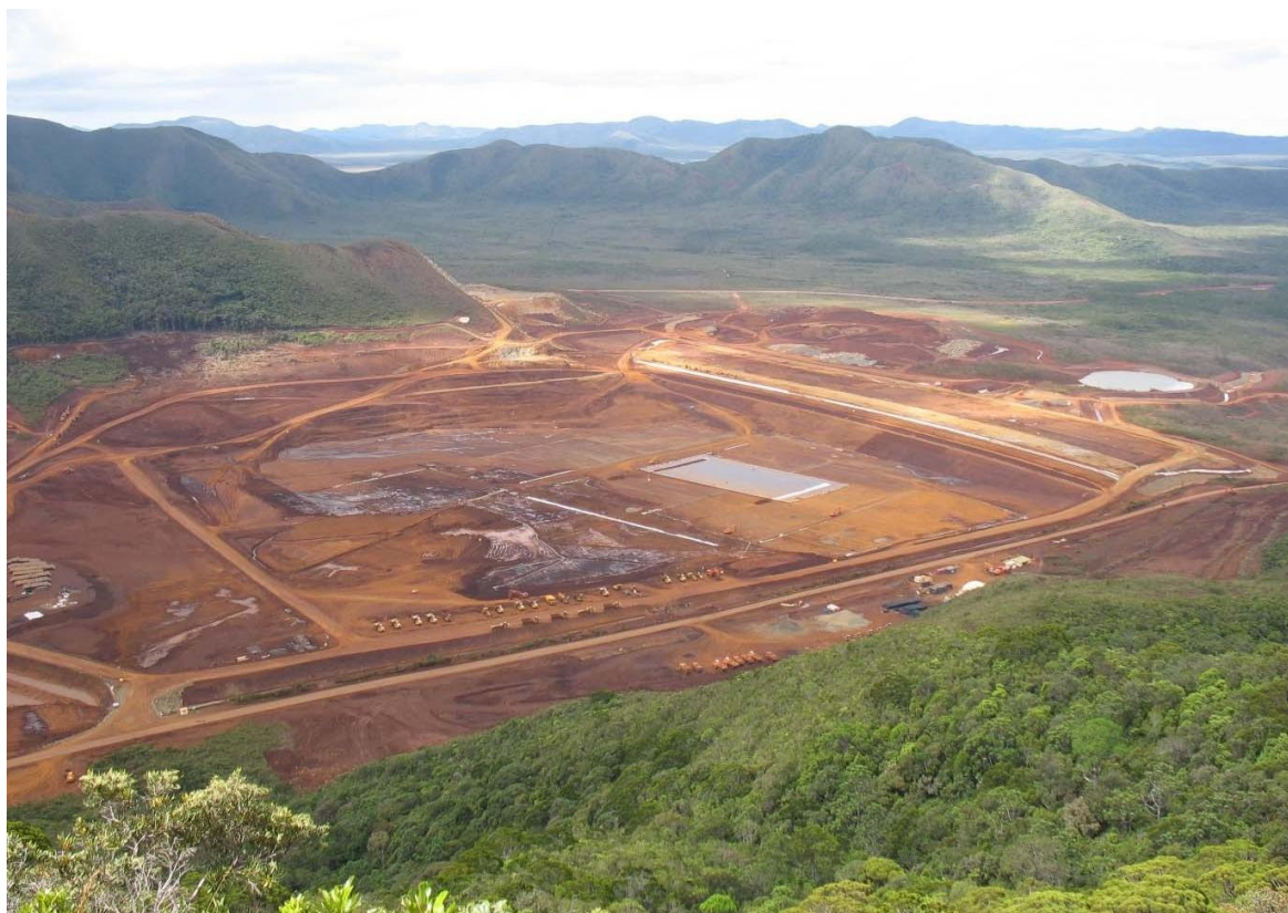
Figure 4. Early stage of construction.
