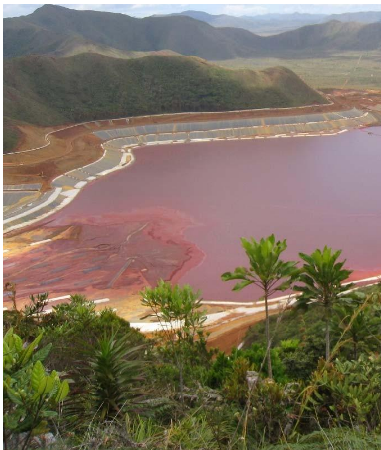
Figure 5. Ballast along slope toe. Storm Water Drainage
