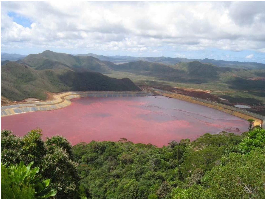
Figure 8. Completed residue storage facility.
