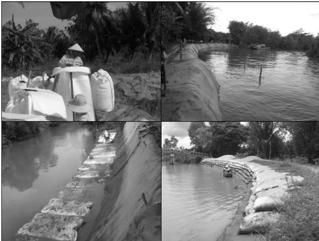
Figure 6: Situation during construction and after completion
