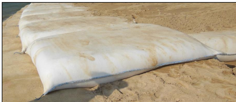
Figure 2. Illustration of a geotextile sand filled container
