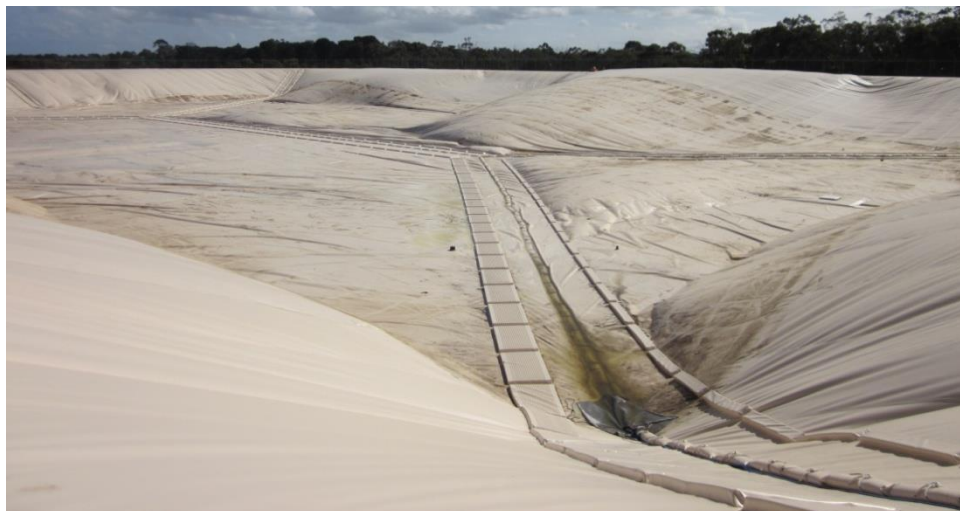
Figure 2. A partially inflated cover with wider floats as walkways on one side of the ballast
