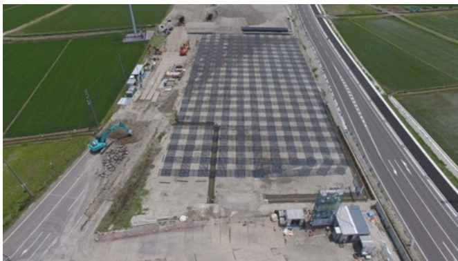
Photo1. Example of geosynthetics laid in grids
