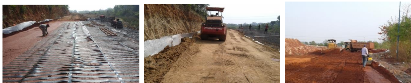
Figure 8. (a) Laying of high strength geogrid and (b) Compaction by vibro-roller (c) Rolling near the wall by baby roller
