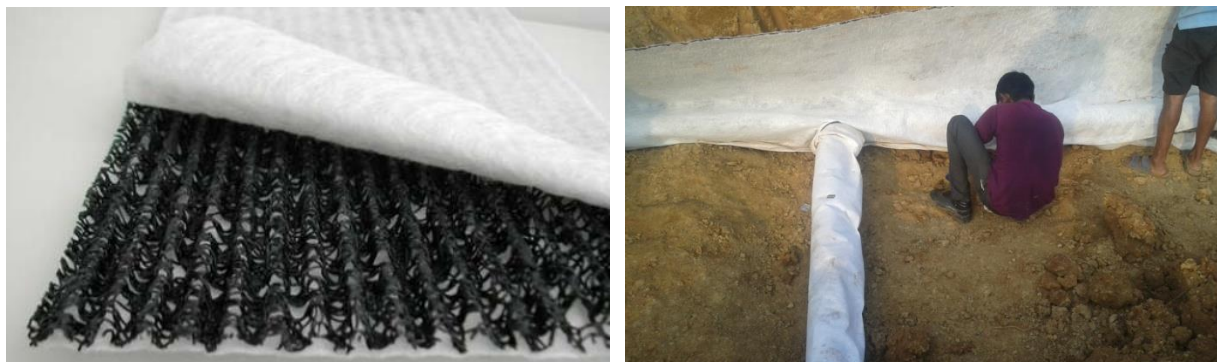
Figure 11 (a) Drainage geo composite and (b) Laying of drainage composite and perforated pipes
