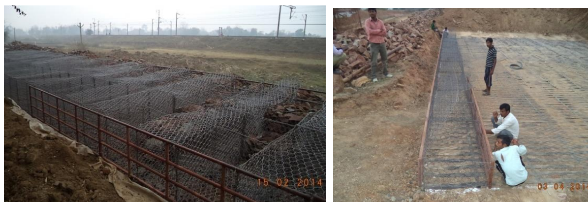
Figure 10. (a) Gabion box laying and Shuttering (b) Laying of Gabion facia with extended bottom with steel wire Drainage measures
