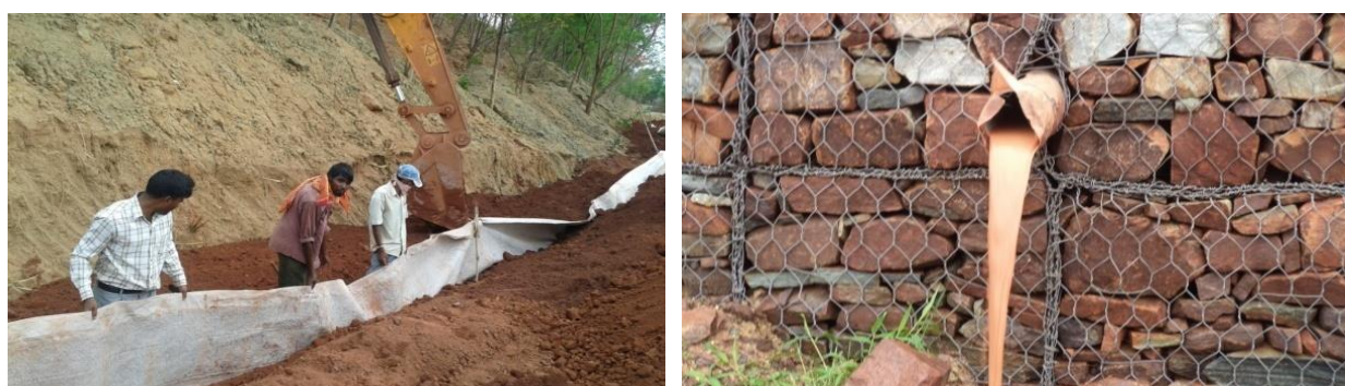
Figure 12 (a) Laying of drainage composite and (b) Proper functioning of drainage composite
