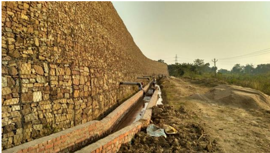
Figure 3 longitudinal drain in front of the wall to collect leachate
