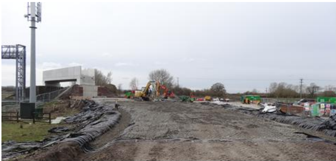
Figure 2. High strength uni-axial geogrid acting as basal reinforcement placed underneath the soil reinforced ramps
