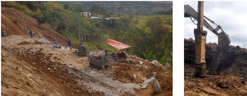
Figure 9. Jet grouted piles and stone columns construction photos
