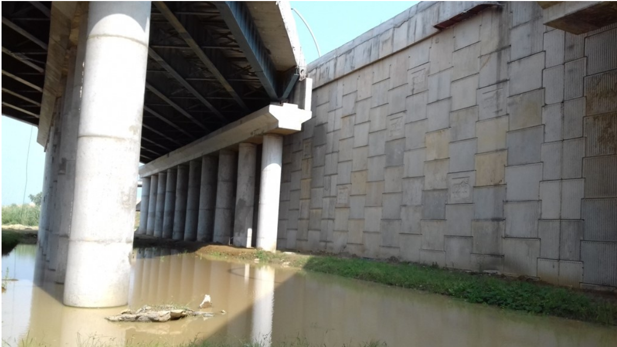
Figure 10 Completed RS wall structure
