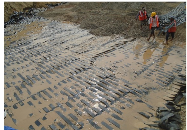
Figure 5 Ground improvement-Laying of Paralink
