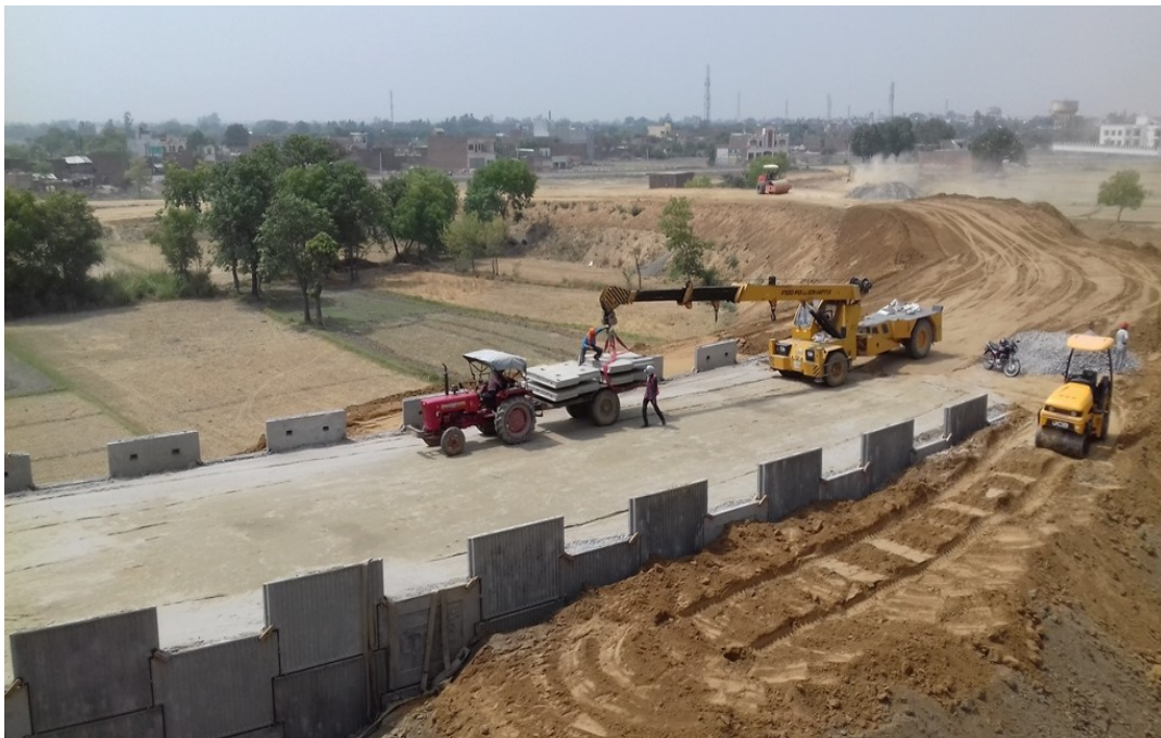
Figure 9 Construction in Progress
