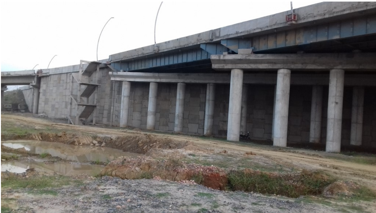
Figure 11 Completed RS wall structure
