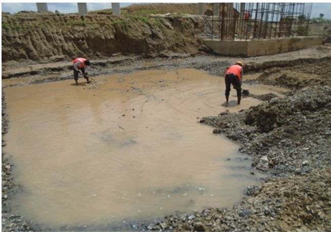
Figure 4 Ground improvement-Excavation in progress
