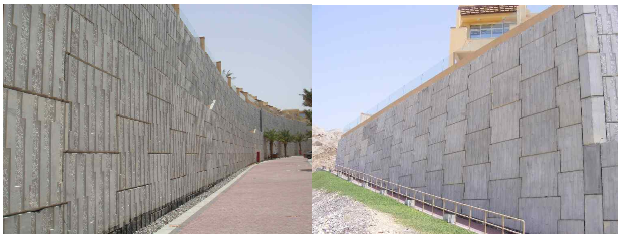
Figure 1. Views of Retaining Wall
