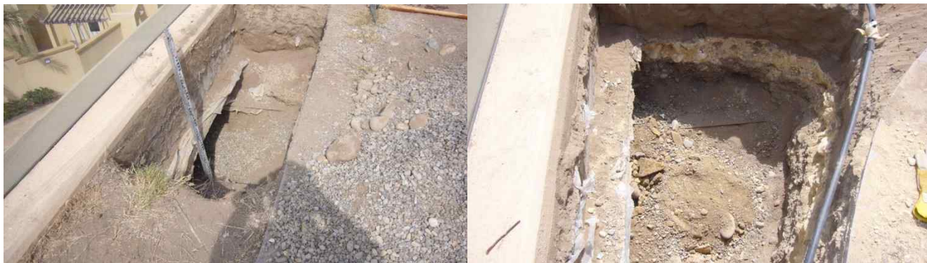
Figure 5: Trial pit excavation
