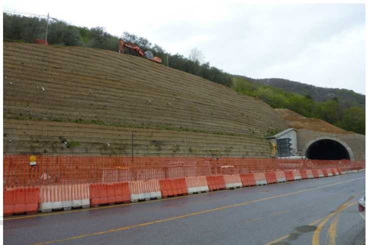
Figure 7. Design cross section and view of the wall at the Southern round-about during construction
