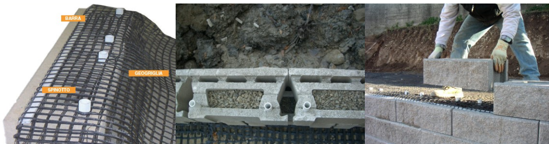
Figure 11. The segmental concrete block facing system with the plastic pins and the groove for connector bars
