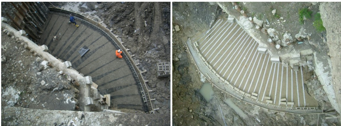
Figure 12. Geogrids being connected to concrete blocks (right); geocomposite drainage strips (left)
