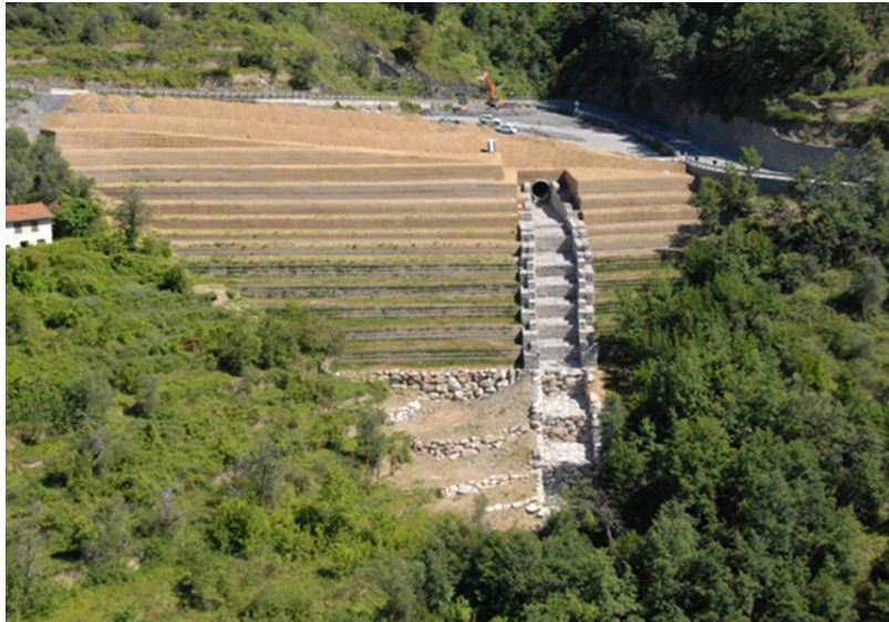
Figure 5. The completed wall with the gabion channel and the plan view of the Acquetico round-about
