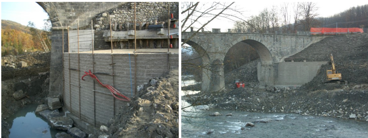
Figure 13. The concrete block facing and the almost completed downstream wing wall
