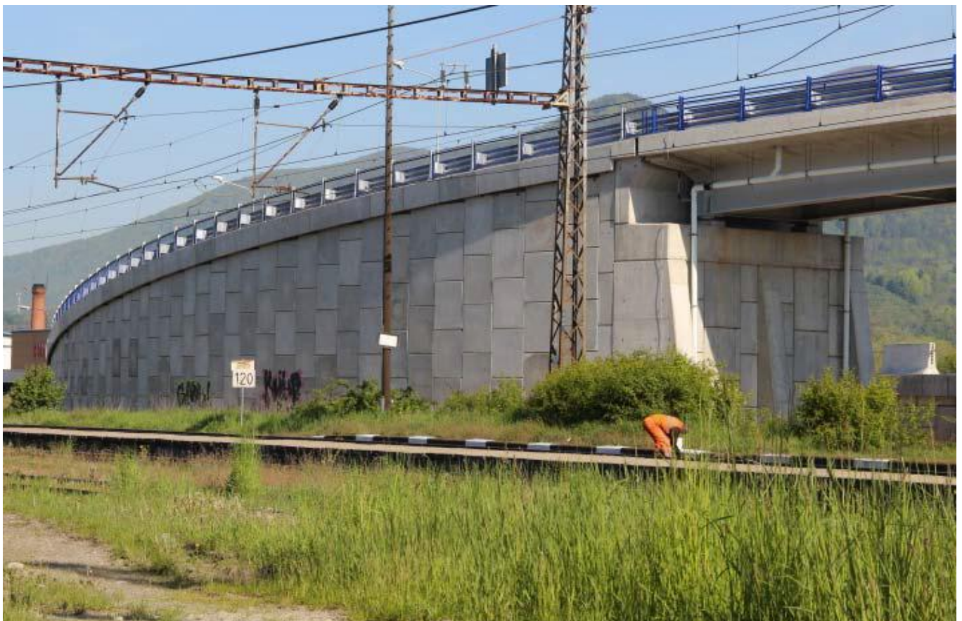
Figure 7. Reinforced soil structure with concrete facing panels adjacent to the railway
