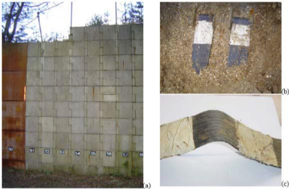
Figure 1. (a) Elevation of TRL experimental Wall with polymer reinforcement ParaWeb, Sample exhumed March 2005 (b) before removal, (c) after removal.
