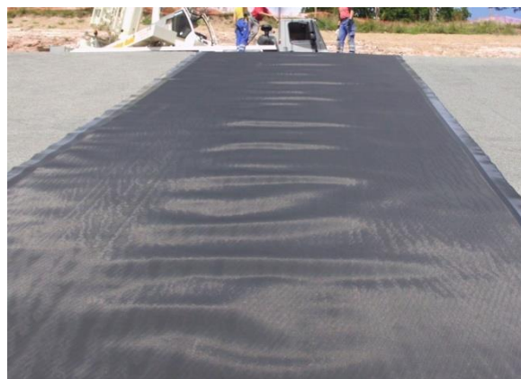
Figure 1. Dimensional stability in the extrusion direction measured along the width of the GMB (left). Intrinsic waviness of the GMB after deployment on the installation site (right).
