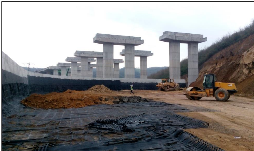
Figure 7. Lapping wall construction behind the concrete retaining wall
