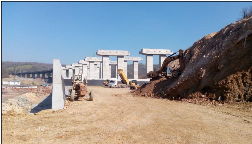
Figure 6. Concrete retaining wall and lapping wall foundation preparation
