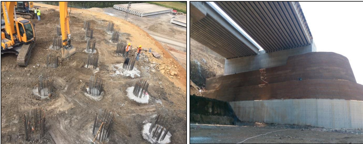
Figure 9. Bored piles and completed green terramesh retaining wall
