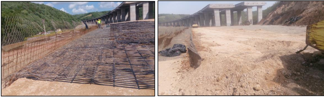
Figure 8. Some stage of green terramesh construction
