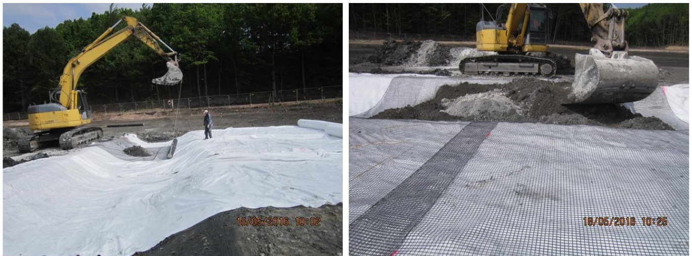
Figure 7. Fixing geosynthetic in the anchor trench.
