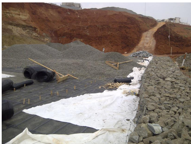
Figure 5: Slope Reinforcement Construction Process (2)
