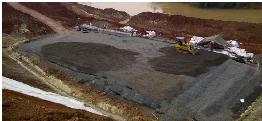
Figure 4: Slope Reinforcement Construction Process (1)
