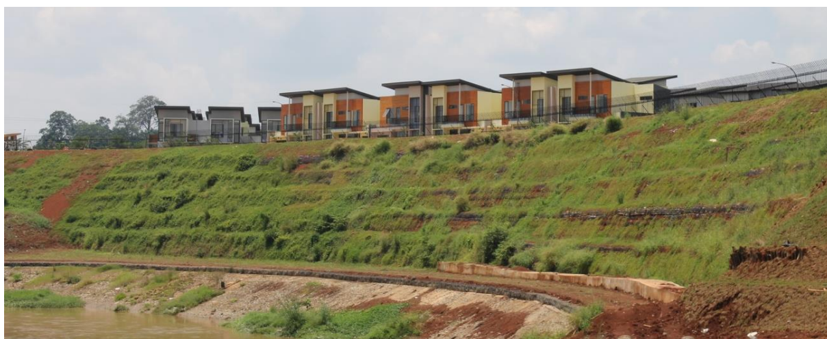
Figure 7: Slope Condition after Construction
