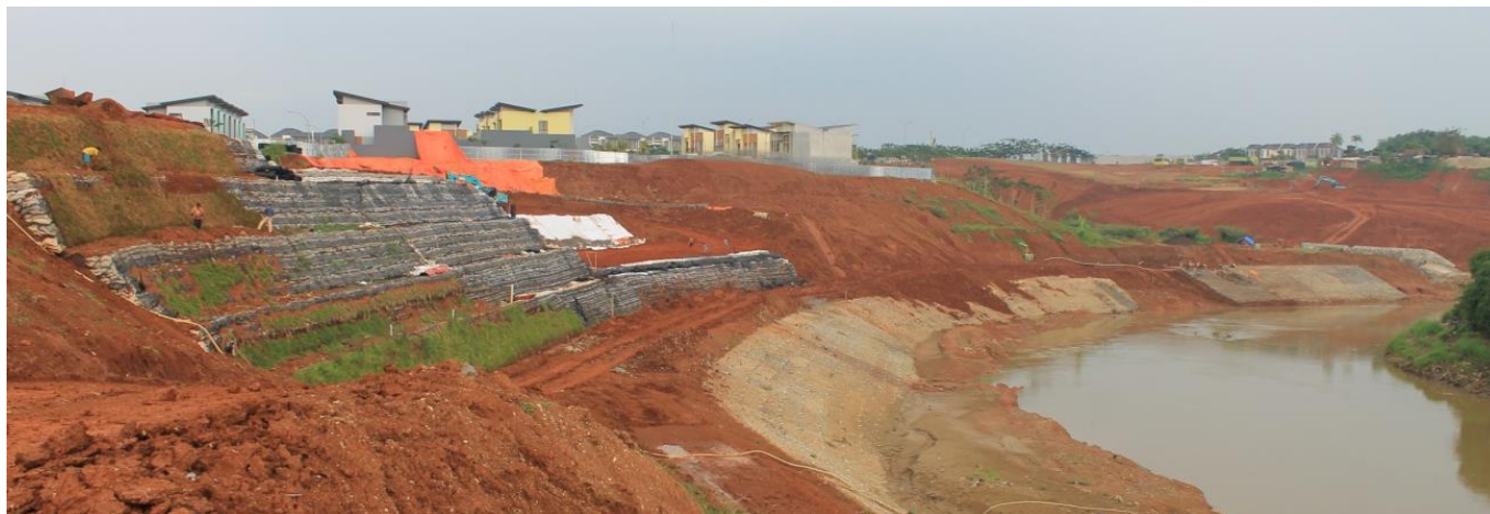
Figure 6: Slope Reinforcement Construction Process (3)
