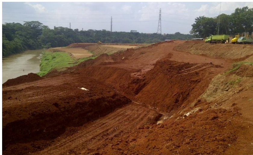
Figure 1: Embankment Slope Existing Condition before Slope Reinforcement Construction
