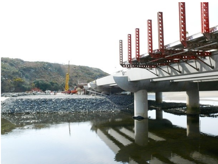
Figure 6. Construction process temporary embankments and permanent causeways
