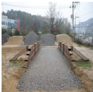
(a) Place and compact the preparatory fill layer
