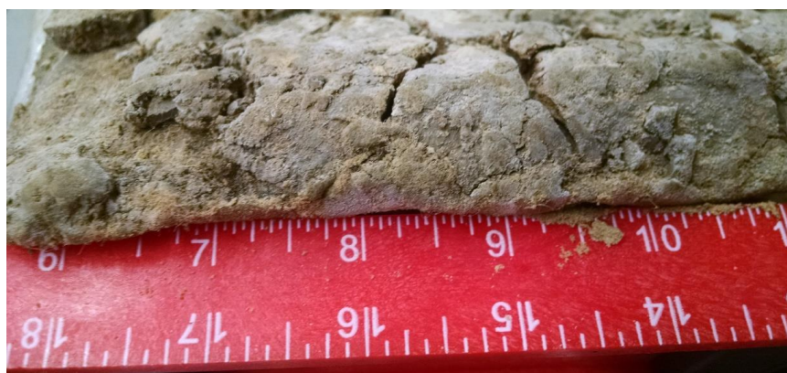
Figure 5. Photograph of accumulated material on upper surface of GCL sample ES-B-1.
