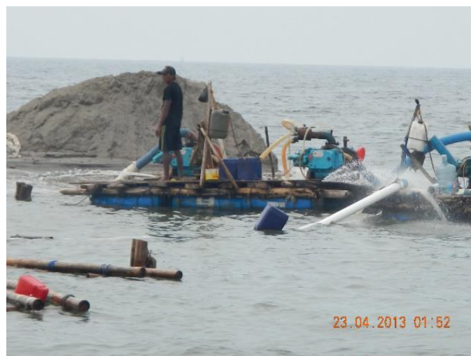
Figure 9 : Sand pumped to the first layer of geotextile tube
