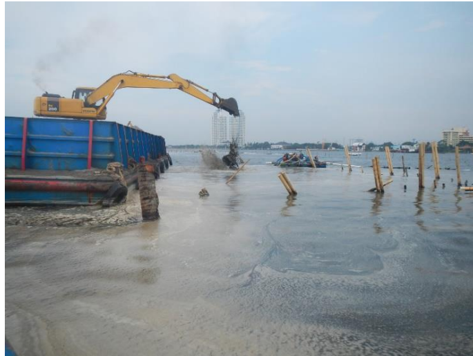
Figure 8 : Sand dumping from barge to stockpile
