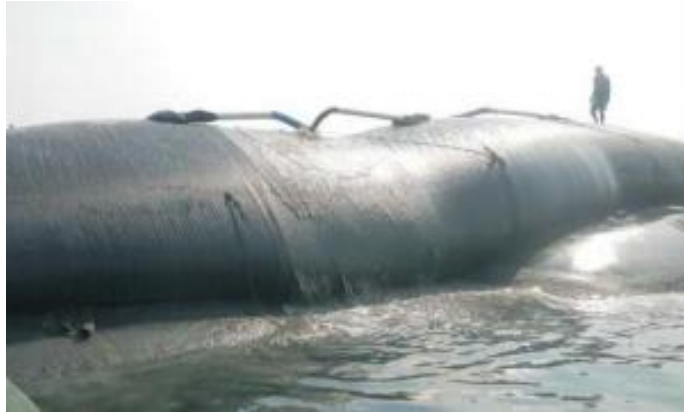
Figure 10 : Geotextile Tube filling process
