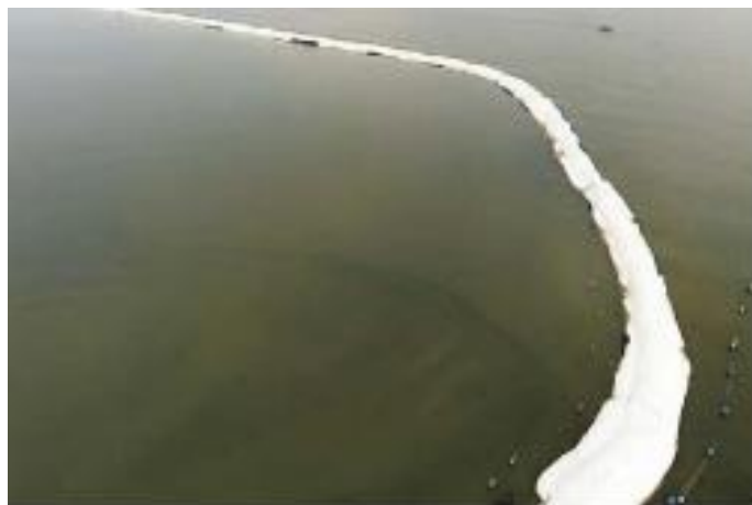
Figure 11 : Geotextile Tube after covered with non woven geotextile
