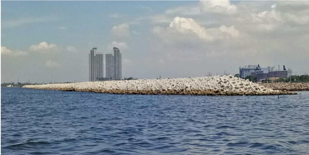
Figure 72 : Geotextile tube condition after protected by armor
