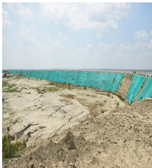
Figure 8. Construction progress at site
