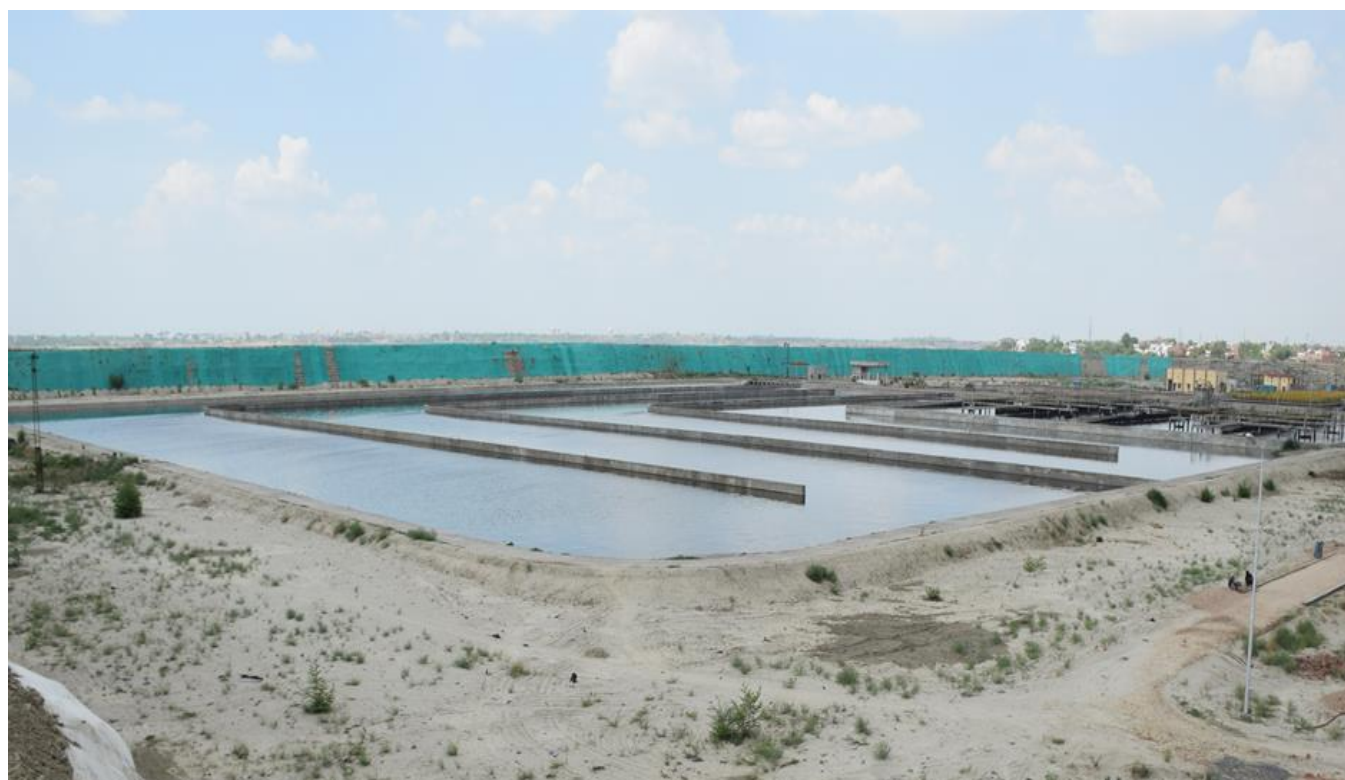
Figure 9. Completed view of Flood protection dyke from the STP
