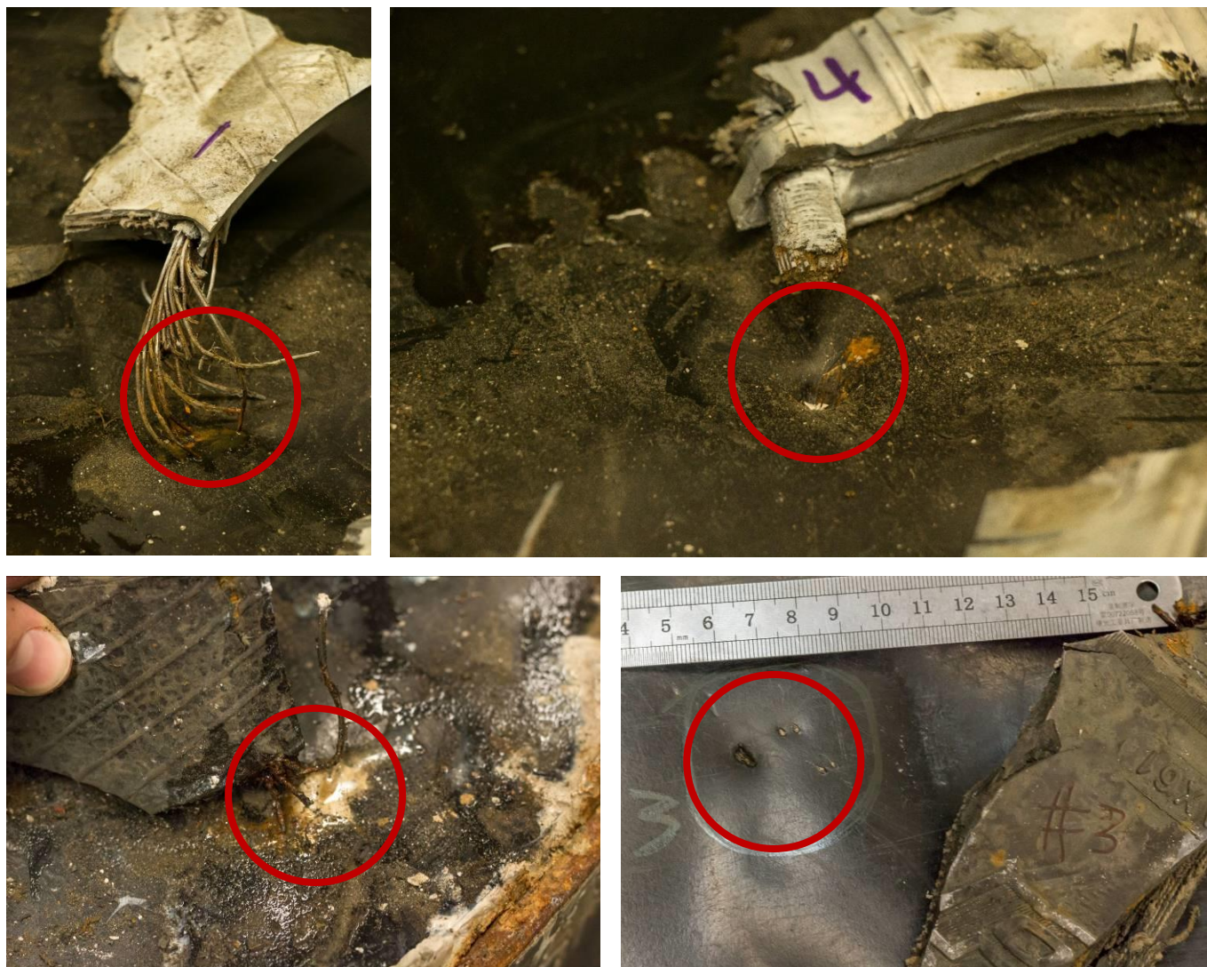
Figure 5: Examples of puncture of geomembrane from TDA (top left = TDA #1; top right = TDA #4; bottom left = unknown; bottom right = TDA #3)
